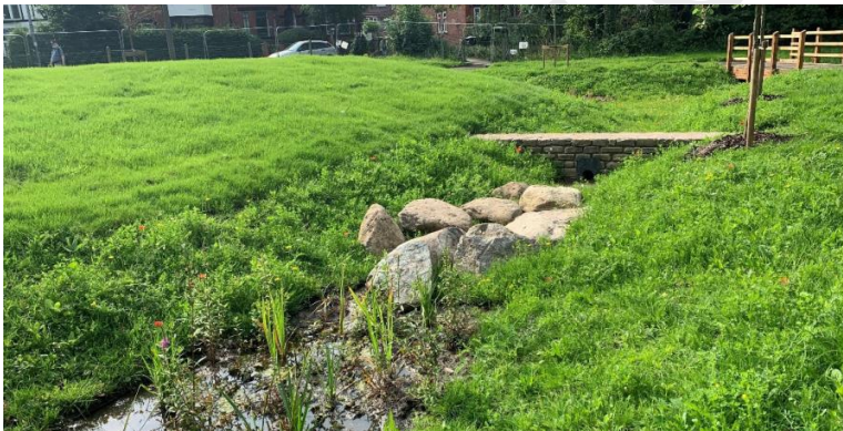
Fig. 5 - Main swale and check dam flow control feature, showing wetland planting and boulders placed to remove energy from circulating flows.
